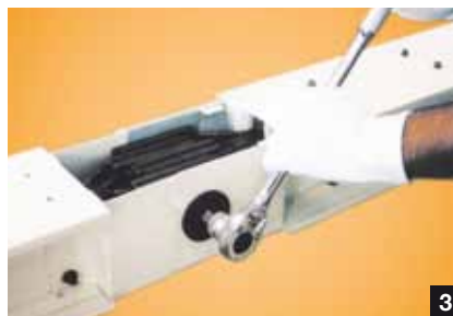
Tighten the "MF" nut by special ratchet wrench till the neck part of the nut is broken and locked.
